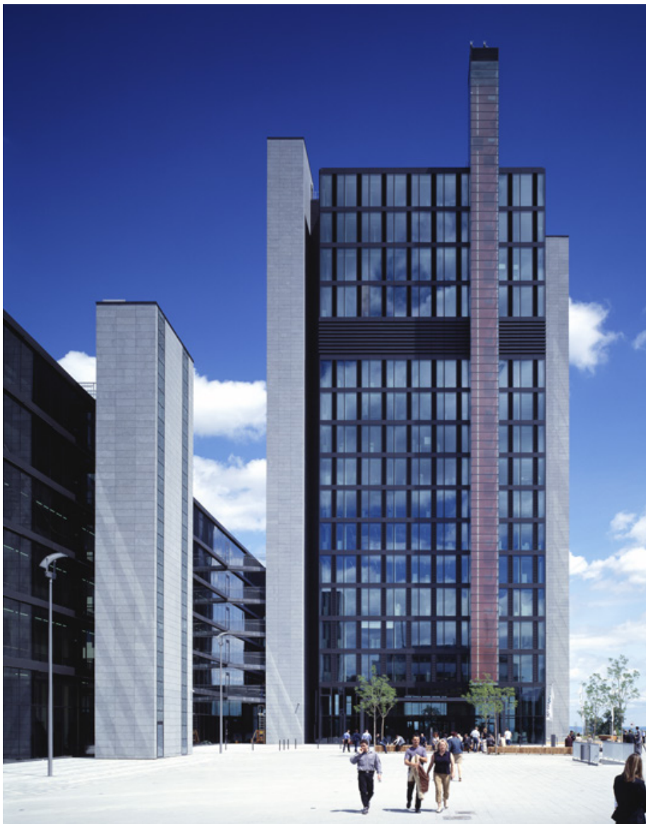
Figure 13. Debitel Headquarters tower with solar chimney.
